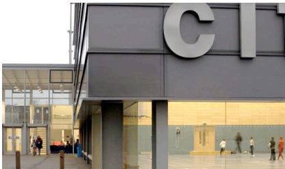
City Academy Bristol - Sports Hall Feilden Clegg Bradley Studios
